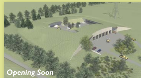
The new Forks Township Public Works Building incorporates a green roof, geothermal heating and cooling, rainwater harvesting / bioswales, passive air preconditioning system, solar site lighting, LED lights, and solar hot water heating.
