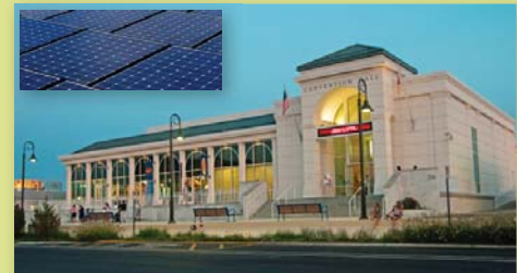
The new Cape May Convention Hall incorporates solar panels on the roof and geothermal heating / cooling to meet LEED Silver guidelines.
